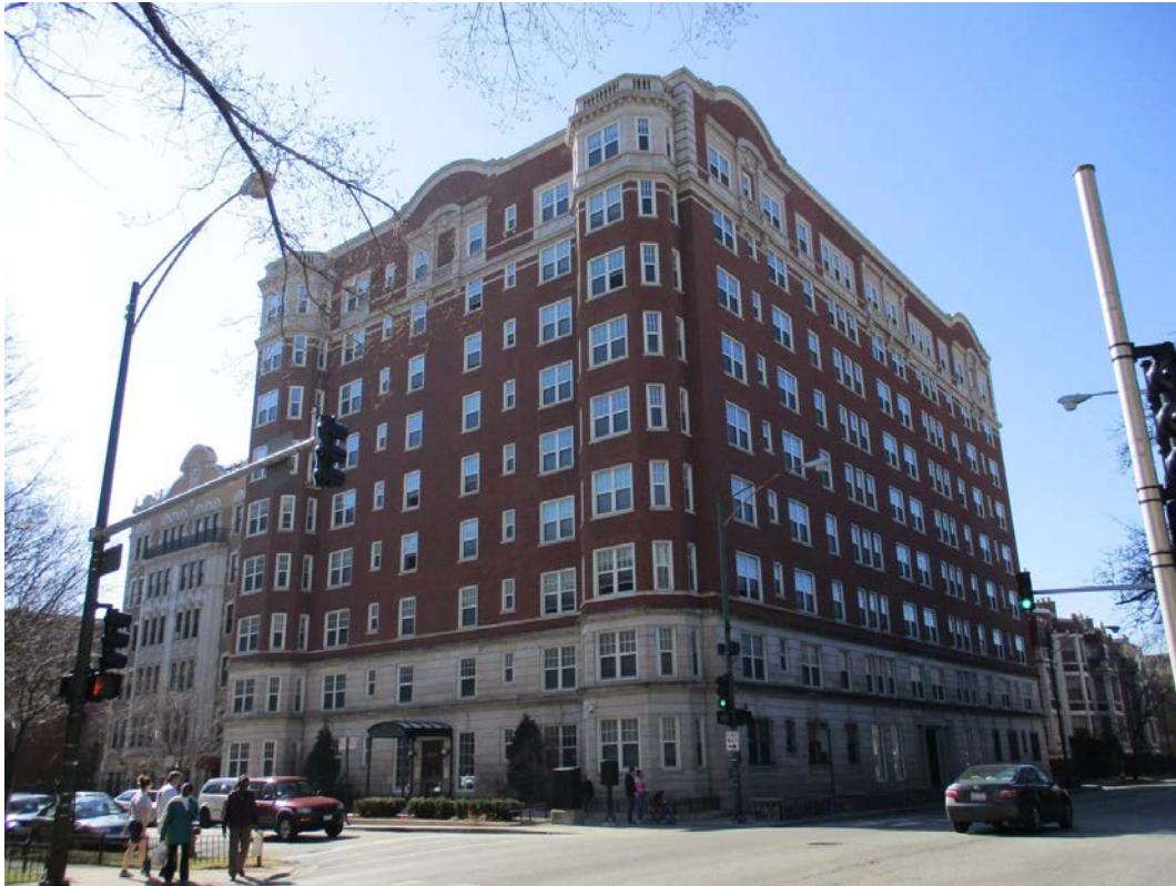
1039 W. Hollywood Avenue/ 5650 N. Kenmore Avenue, view looking southwest from W. Hollywood Avenue toward East and North facades
