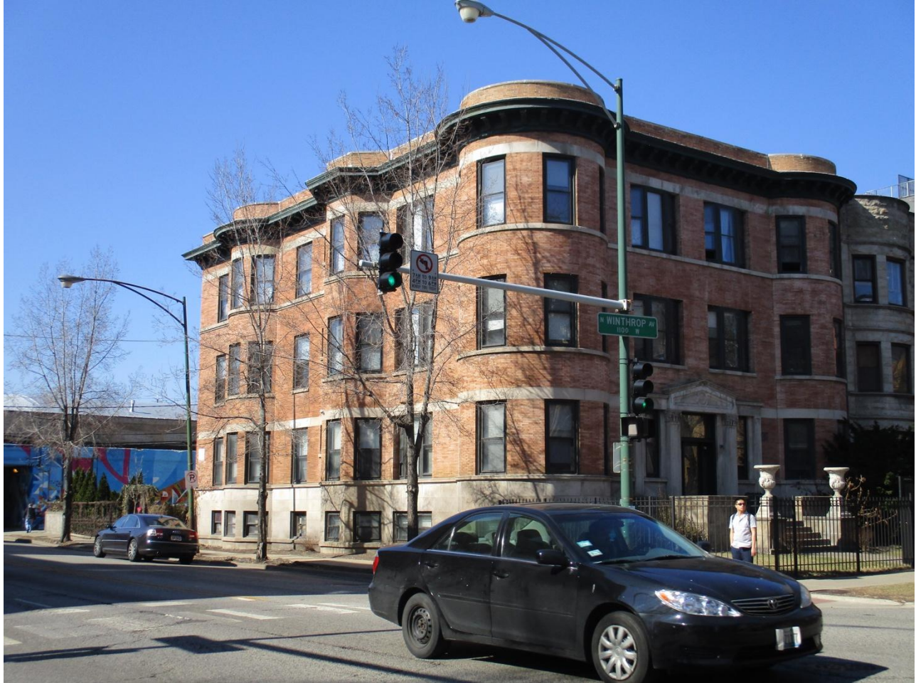
5700 N. Winthrop Avenue, view looking northwest from W. Hollywood Avenue toward South and East facades
