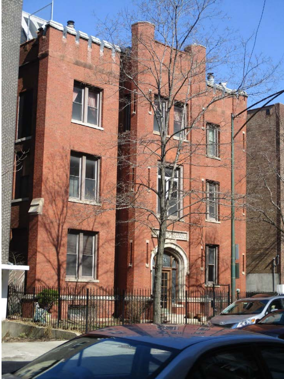
1054 W. Hollywood Avenue, view looking northeast from W. Hollywood Avenue toward South facade
