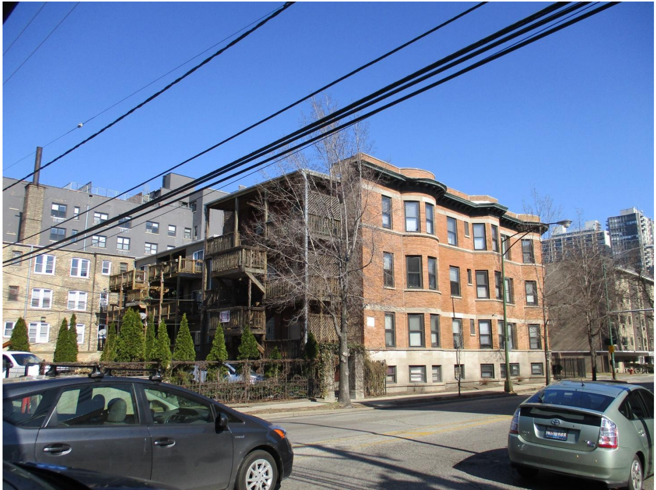
5700 N. Winthrop Avenue, view looking northeast from W. Hollywood Avenue toward South facade
