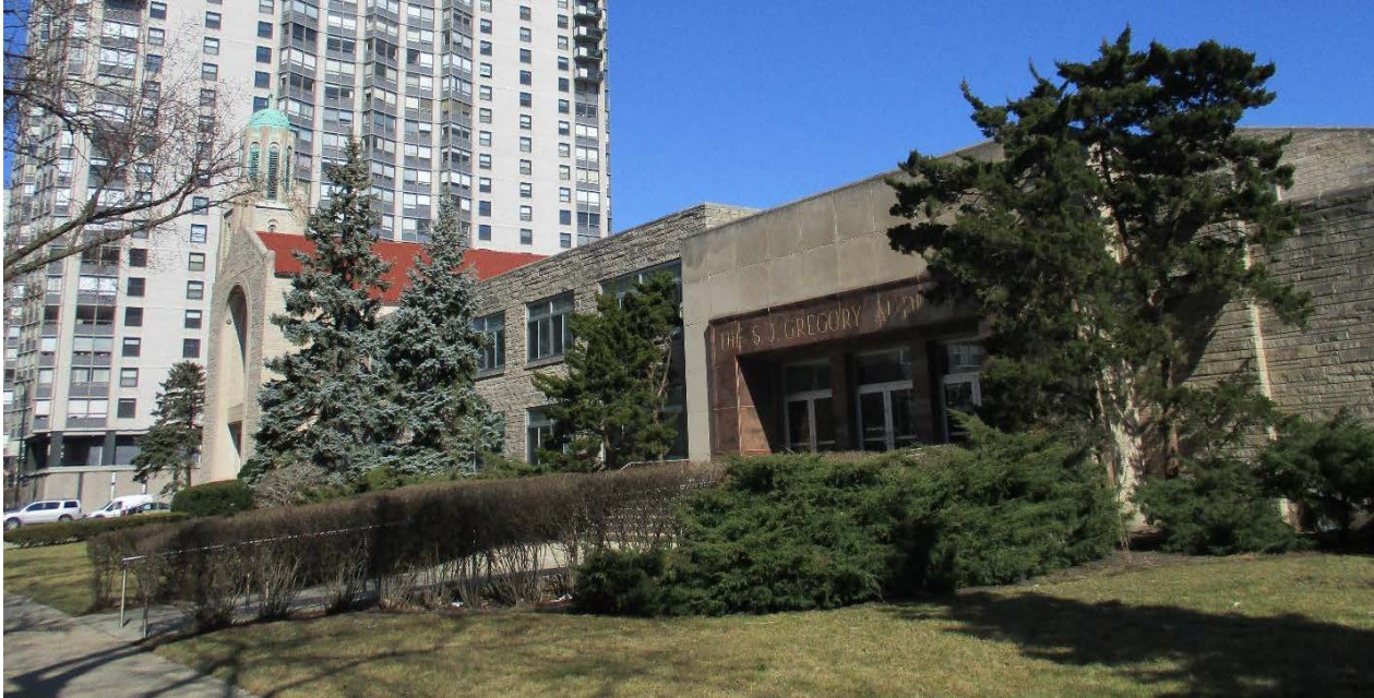
5649 N. Sheridan Road, view looking northeast from N. Sheridan Road toward West facade of community and educational wing of the church complex
