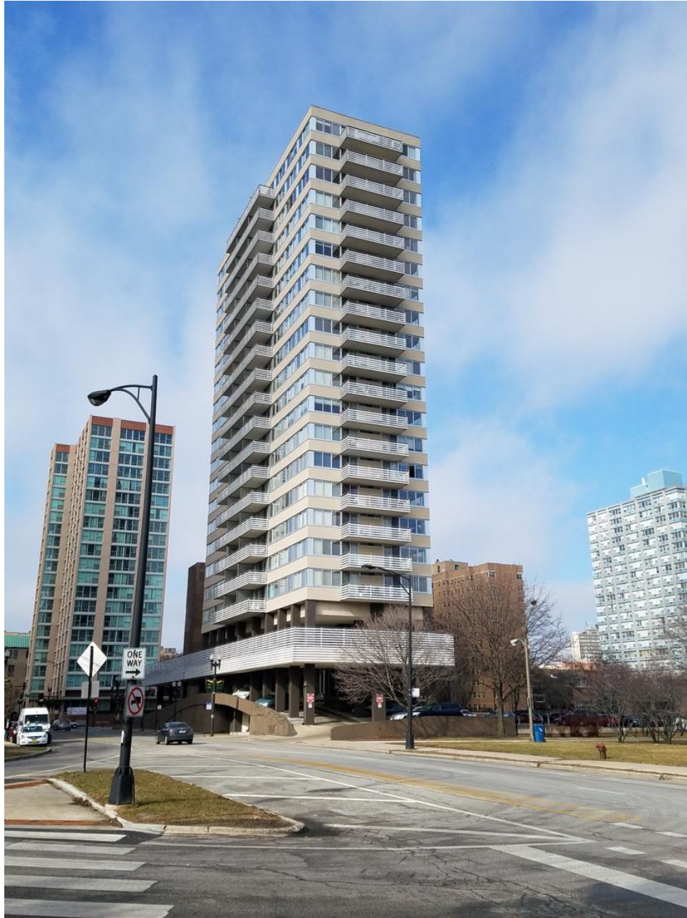
5601 N. Sheridan Road, view looking northwest from W. Bryn Mawr Avenue toward South and East facades
