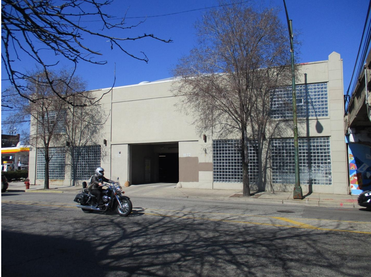
1122 W. Hollywood Avenue, view looking north from W. Hollywood Avenue toward South facade
