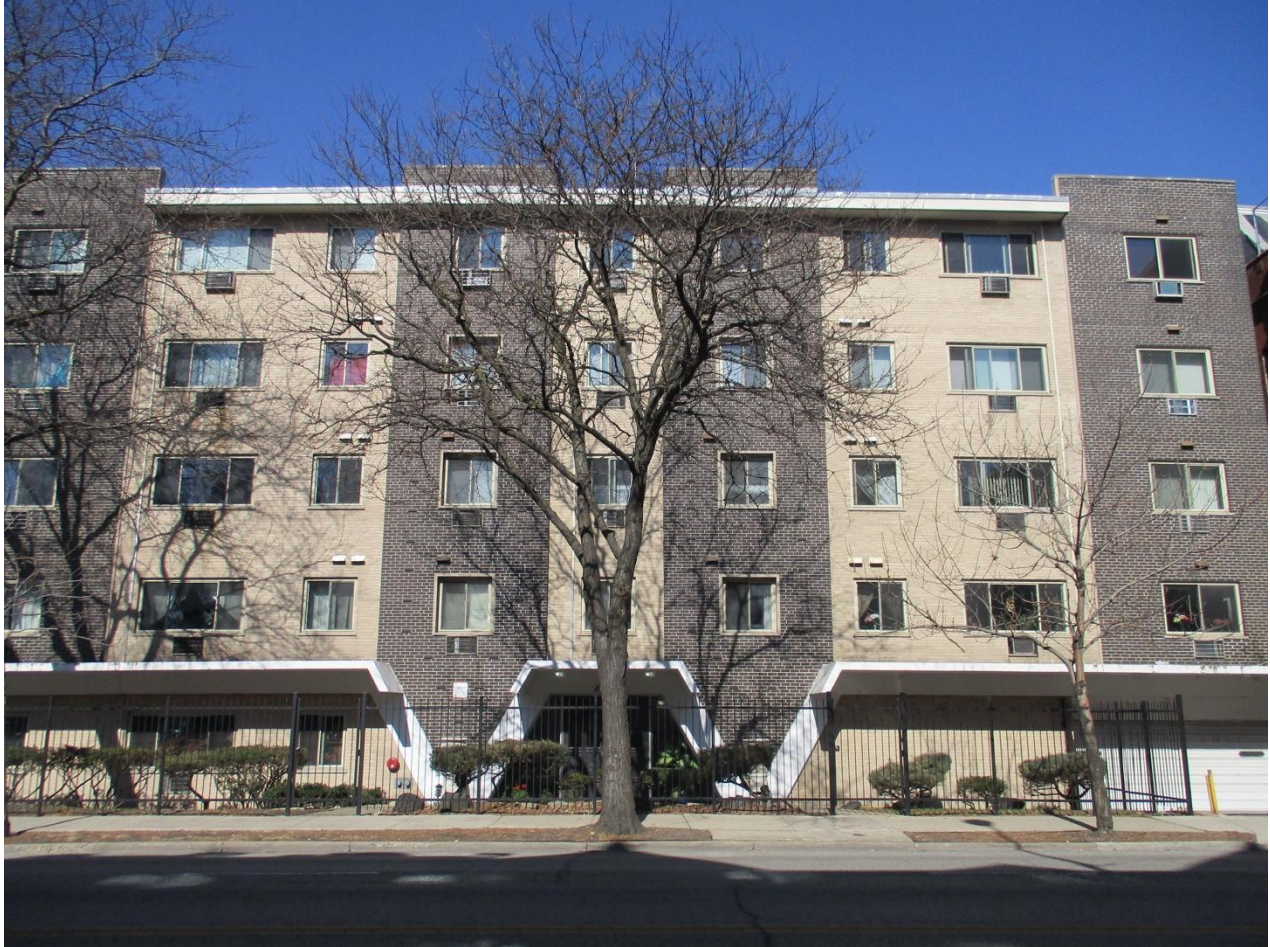
1060 W. Hollywood Avenue, view looking north from W. Hollywood Avenue toward South facade
