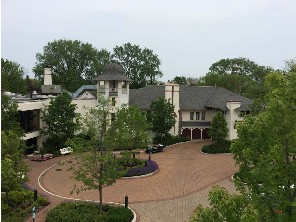
900 W. Foster Avenue, Saddle & Cycle Club, view looking east from parking lot toward main club building
