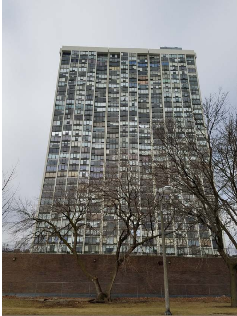
5445-5455 N. Sheridan Road, view looking west from Lincoln Park toward South tower, East facade, with parking structure in foreground
