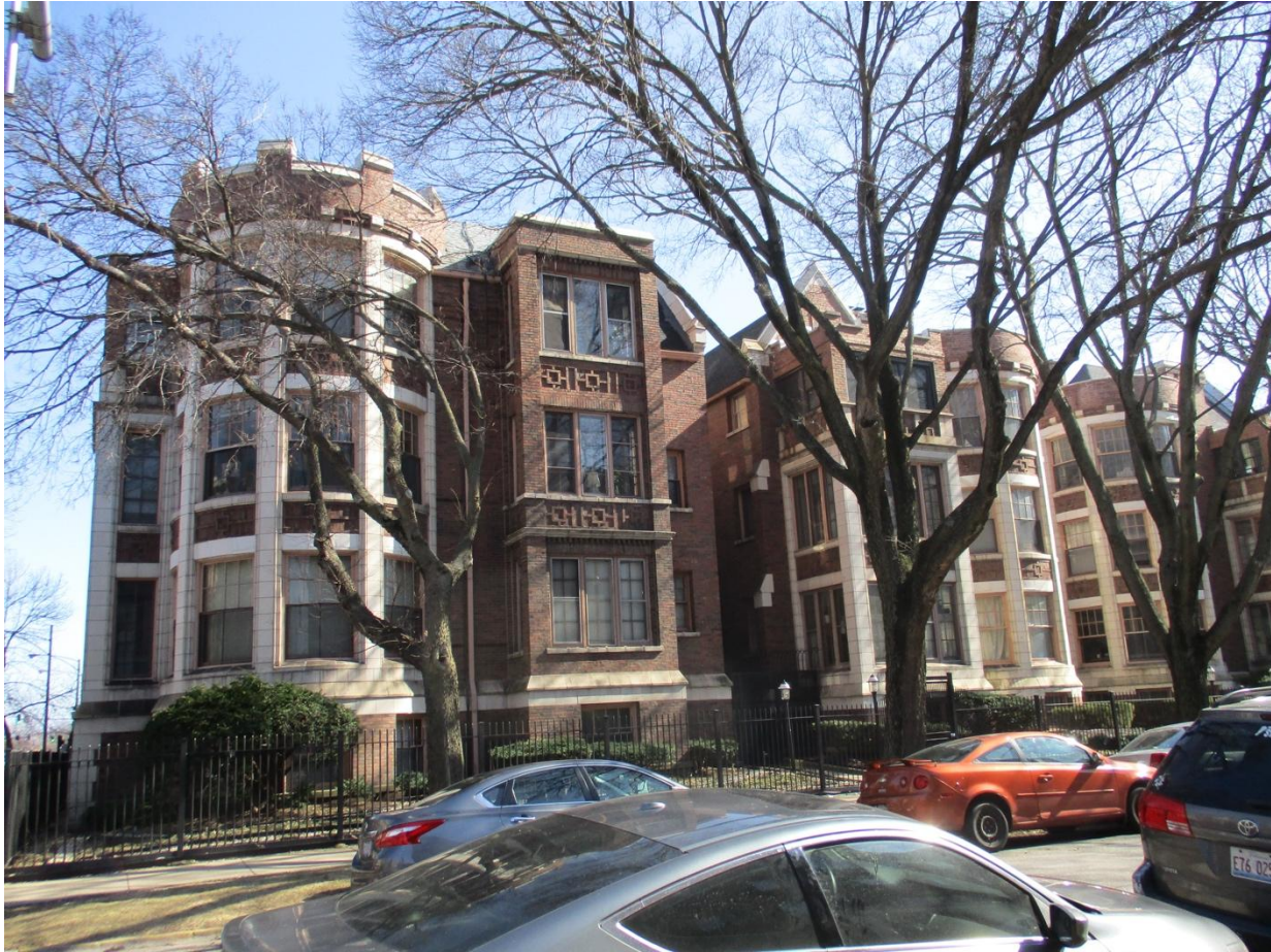
1055-1065 W. Hollywood Avenue / 5641 N. Winthrop Avenue, view looking southeast from N. Winthrop Avenue toward West façade
