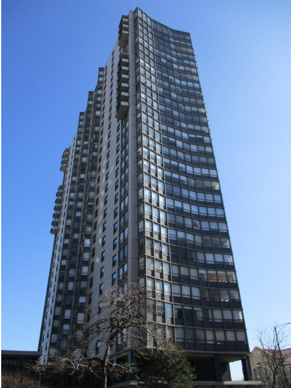
5701 N. Sheridan Road, view looking southeast from N. Sheridan Road, toward North and West facades of South tower
