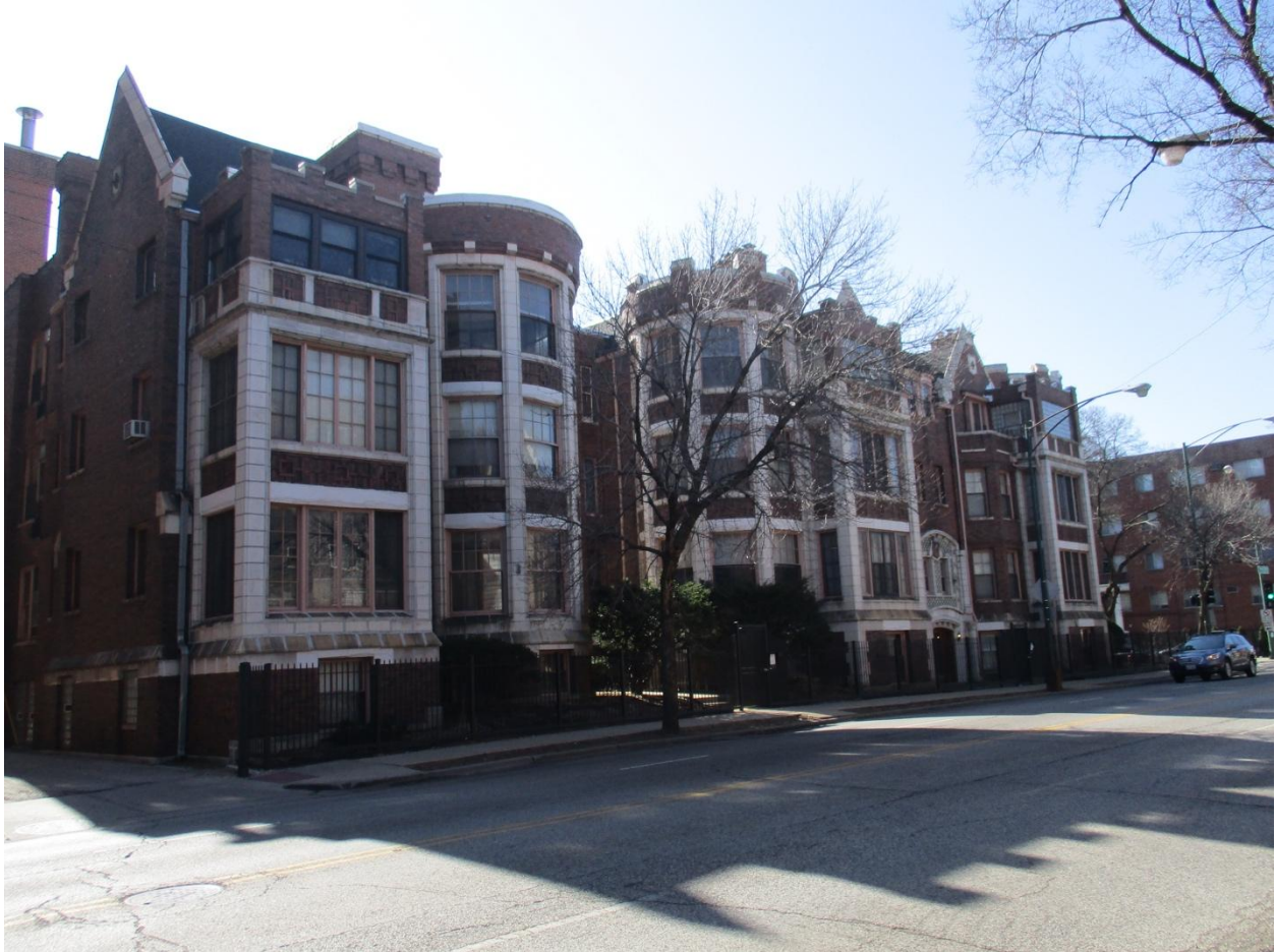
1055-1065 W. Hollywood Avenue / 5641 N. Winthrop Avenue, view looking northwest from W. Hollywood Avenue toward North facade
