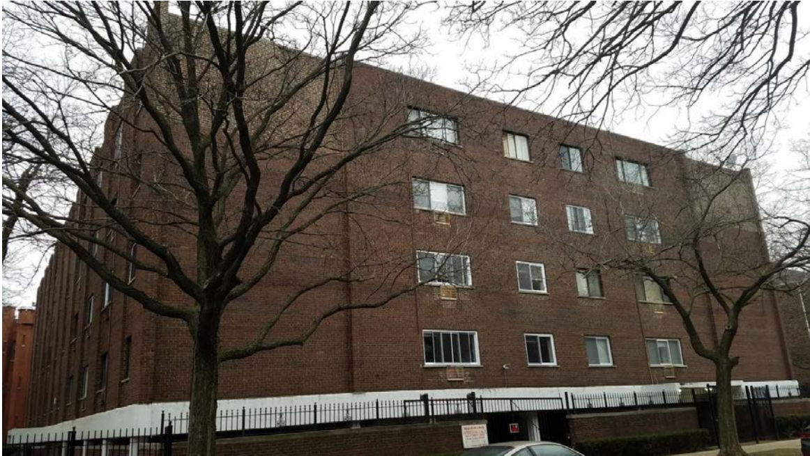
1040 W. Hollywood Avenue, view looking northwest from N. Kenmore Avenue toward South and East facades
