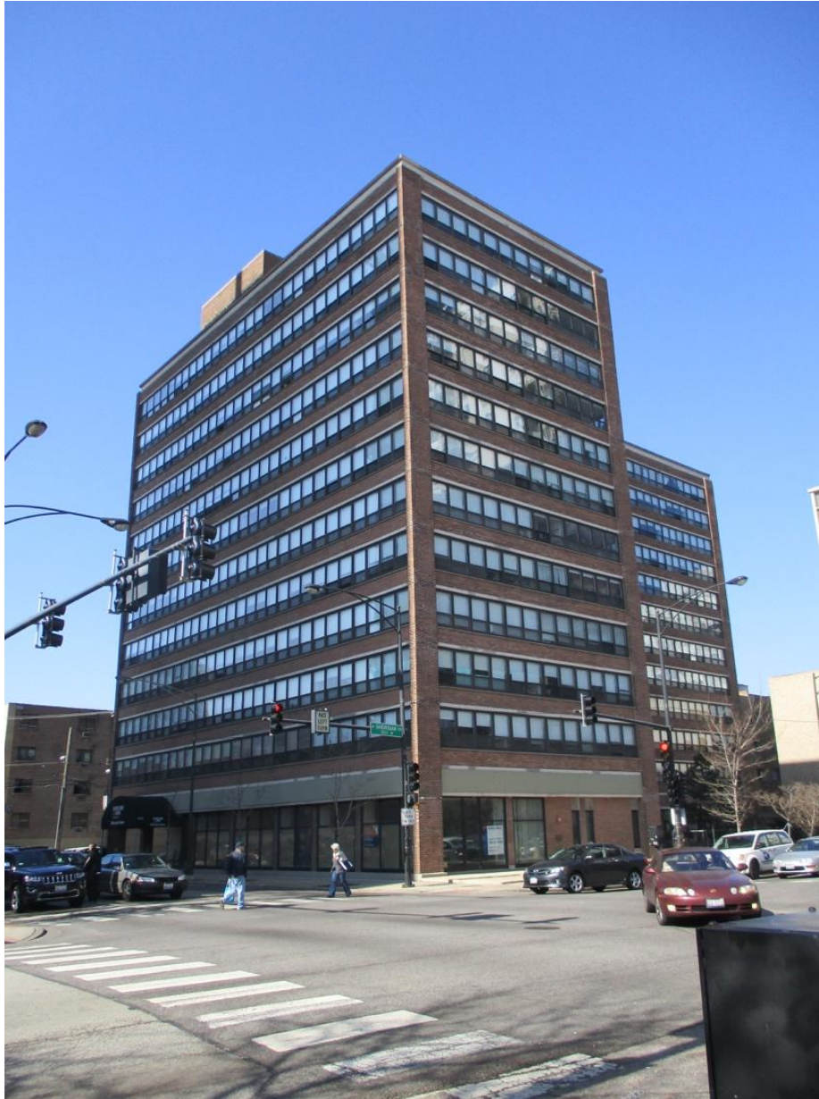
5700 N. Sheridan Road, view looking northwest from N. Sheridan Road toward South and East facades
