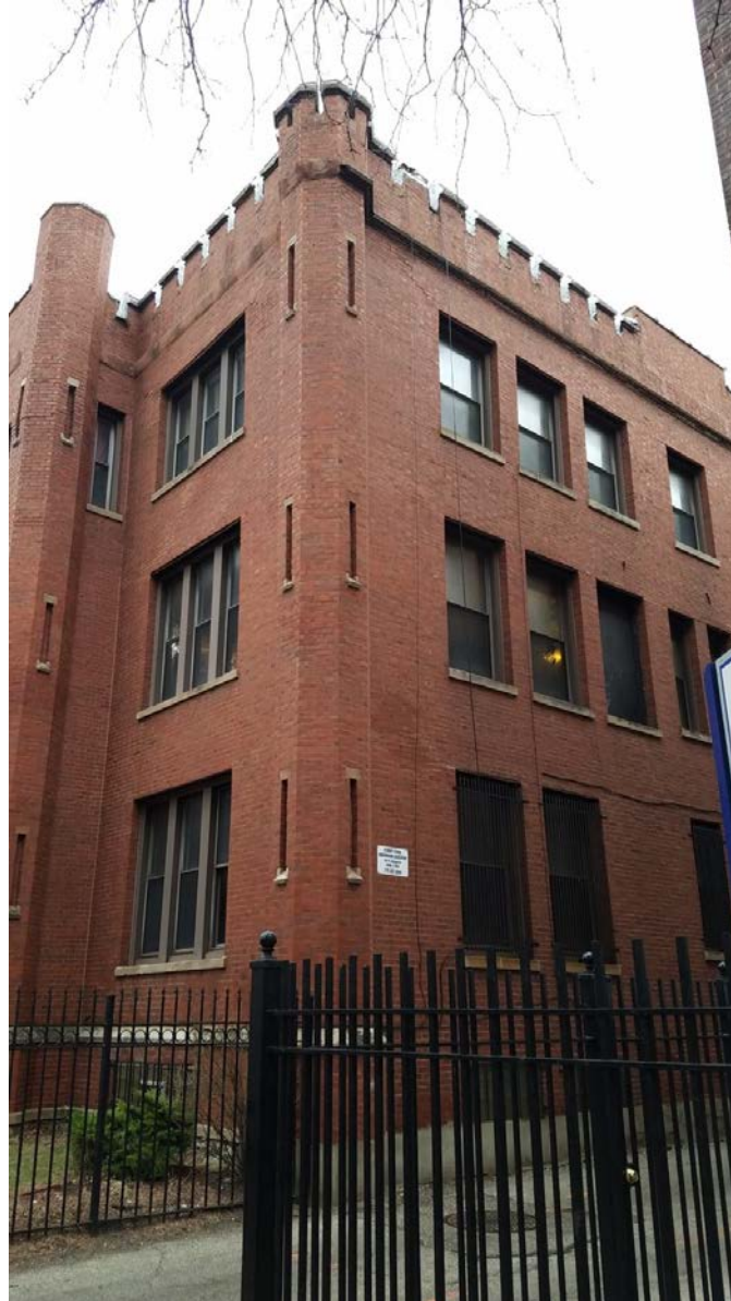
1054 W. Hollywood Avenue, view looking northwest from W. Hollywood Avenue toward South and East facades
