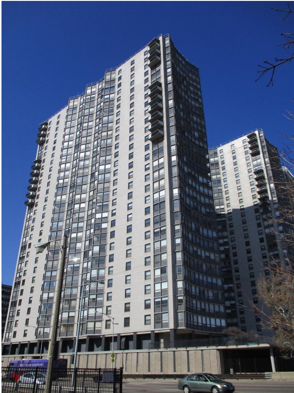
5701 N. Sheridan Road, view looking northwest from W. Hollywood Avenue toward South and East facades of South tower, North tower in background
