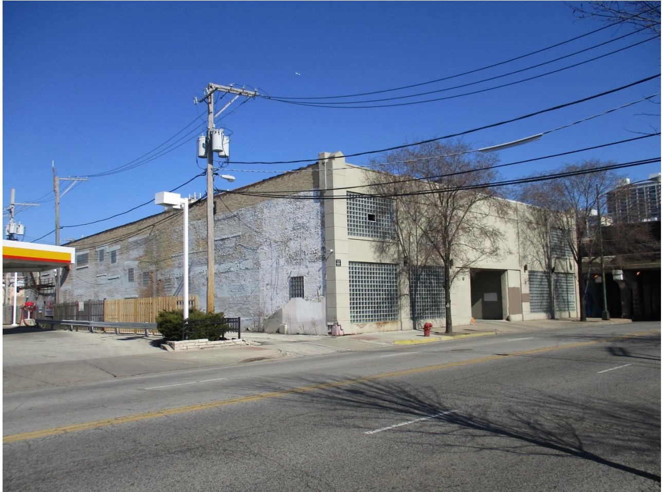
1122 W. Hollywood Avenue, view looking northeast from W. Hollywood Avenue toward West and South facades
