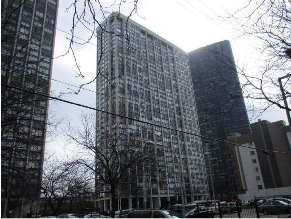
5445-5455 N. Sheridan Road, view looking southeast from N. Sheridan Road toward South tower, North and West facades, with North tower visible on left
