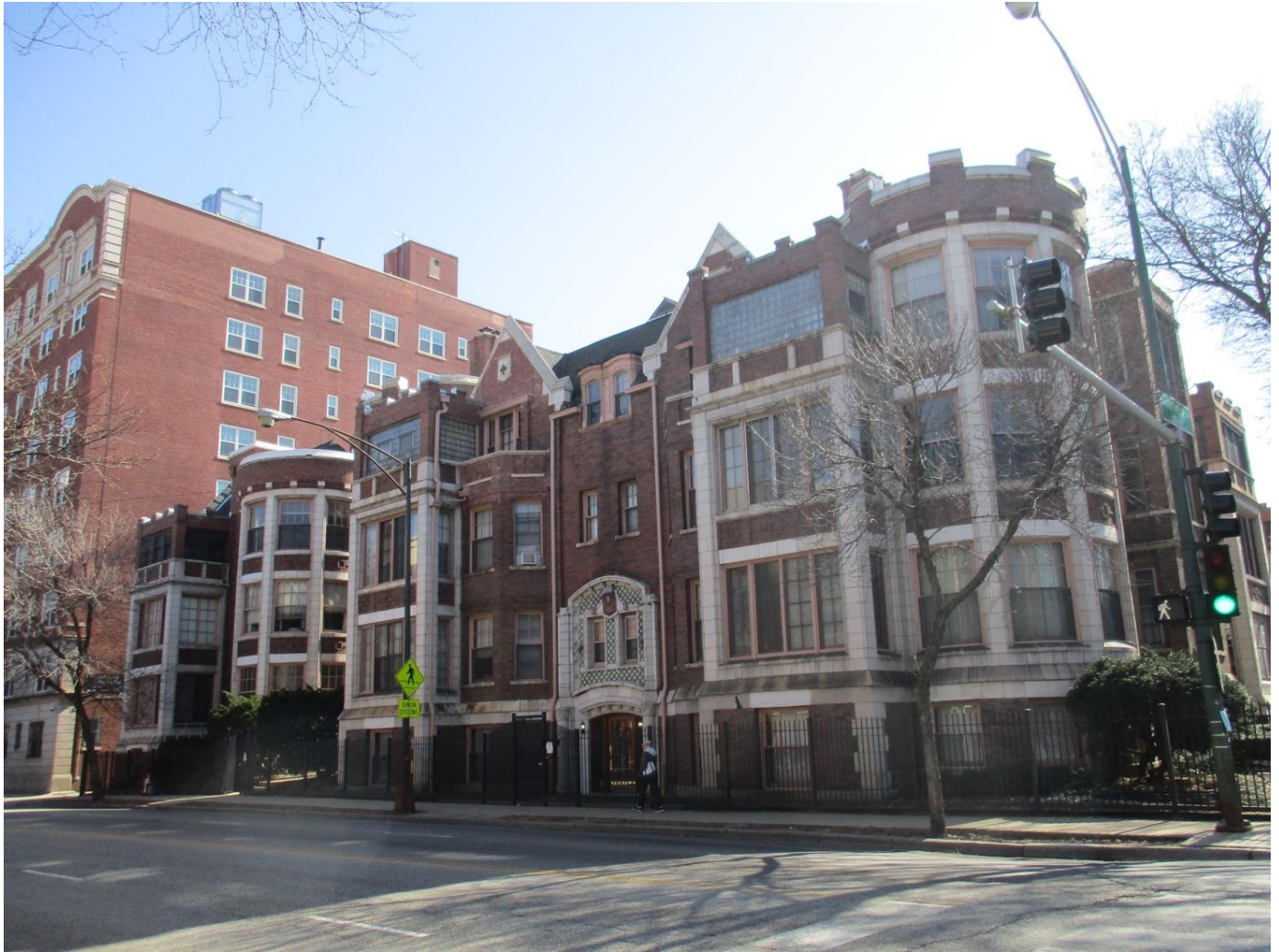
Photo 1 – 1055-1065 W. Hollywood Avenue / 5641 N. Winthrop Avenue
