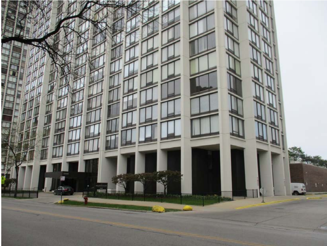
5445-5455 N. Sheridan Road, view looking northeast from N. Sheridan Road toward South tower, detail of ground level support piers
