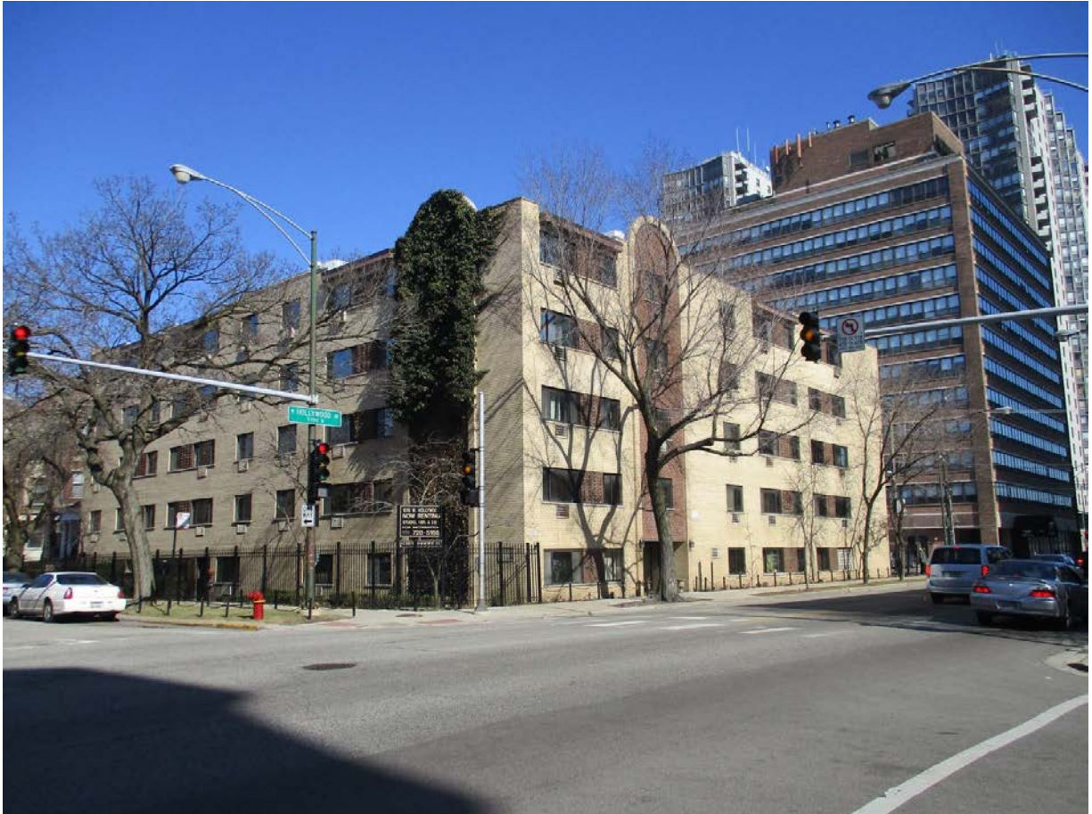
1016 W. Hollywood Avenue, view looking northeast from W. Hollywood Avenue toward South and East facades
