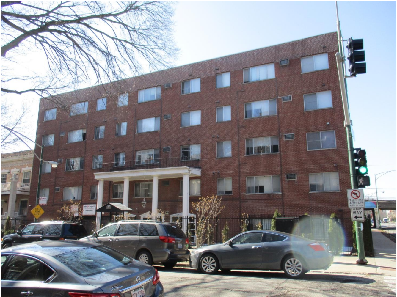
1111 W. Hollywood Avenue, view looking west from N. Winthrop Avenue toward East facade
